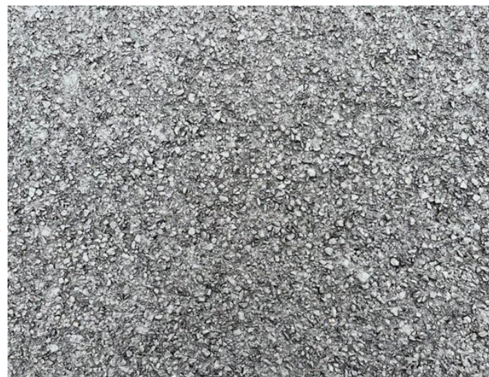
Pictured below: Mat and Double Seal with 78M stone as the top stone. Note the larger sized aggregate as compared to the above picture.
