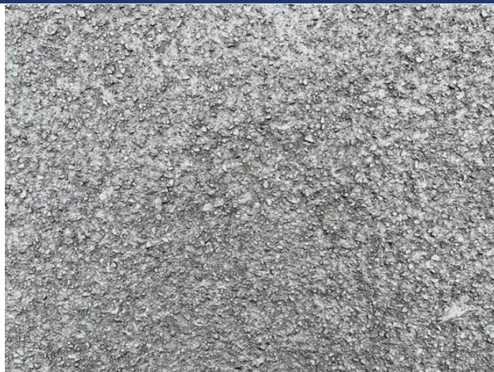
Pictured above: Mat and Double Seal with 14M stone as the top stone.
