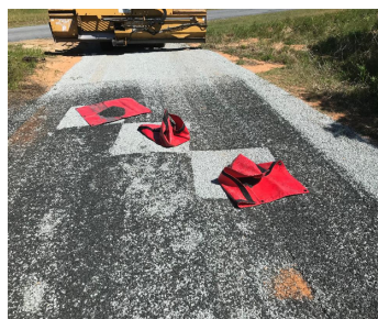
Pictured left: Chip Seal stone spreader calibration.
