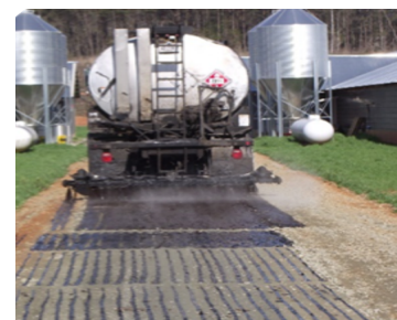
Pictured left: Chip Seal stone spreader calibration.
